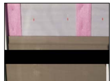
Using Sill Gasket to Create Drainage Plane
